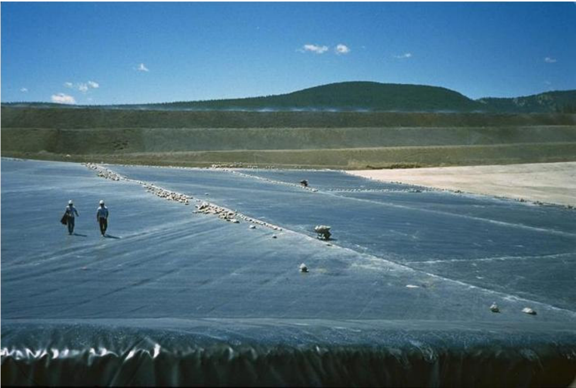
PHOTO 2 – GEOMEMBRANE LINED GOLD HEAP LEACH OPERATION IN MONTANA
