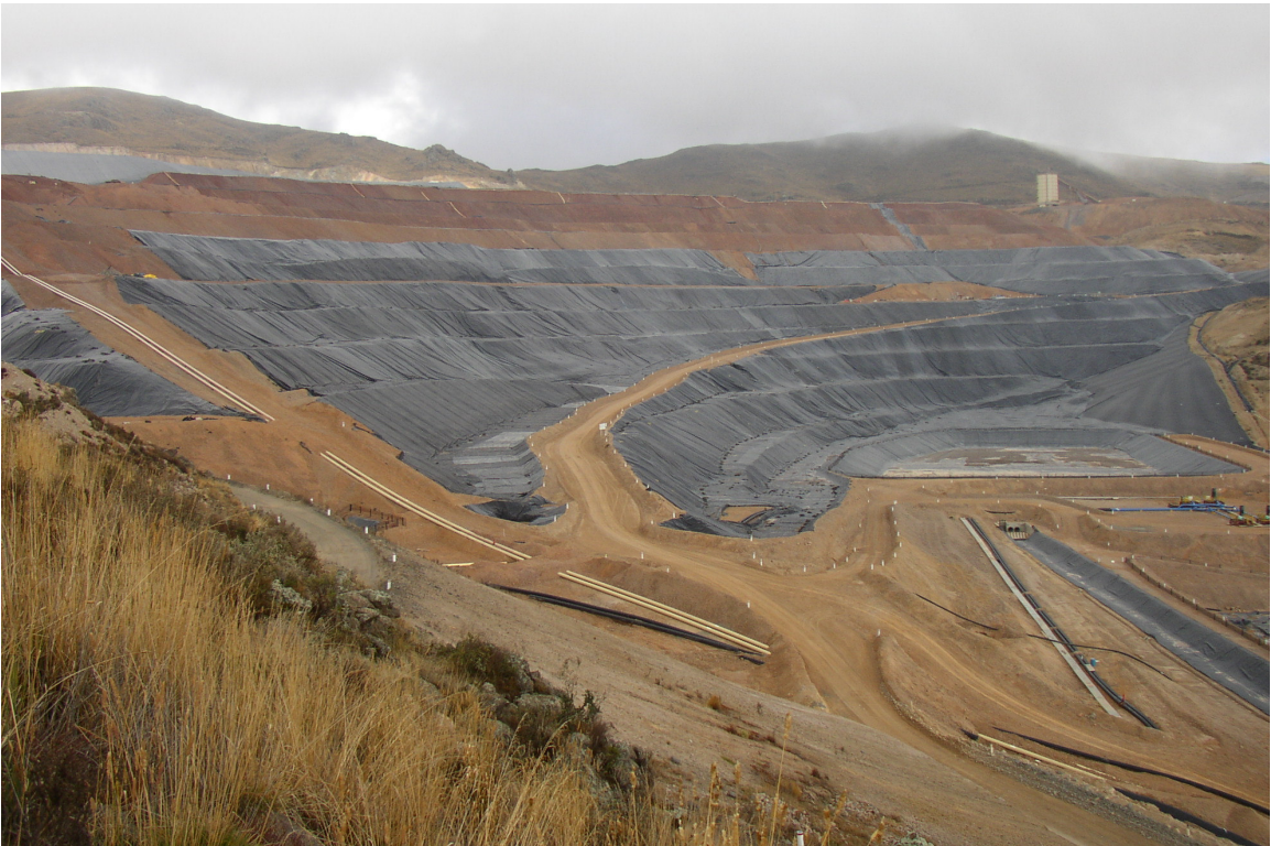
PHOTO 10 – HEAP SLOPE COVERED BY GEOMEMBRANE LINER RAIN COAT
