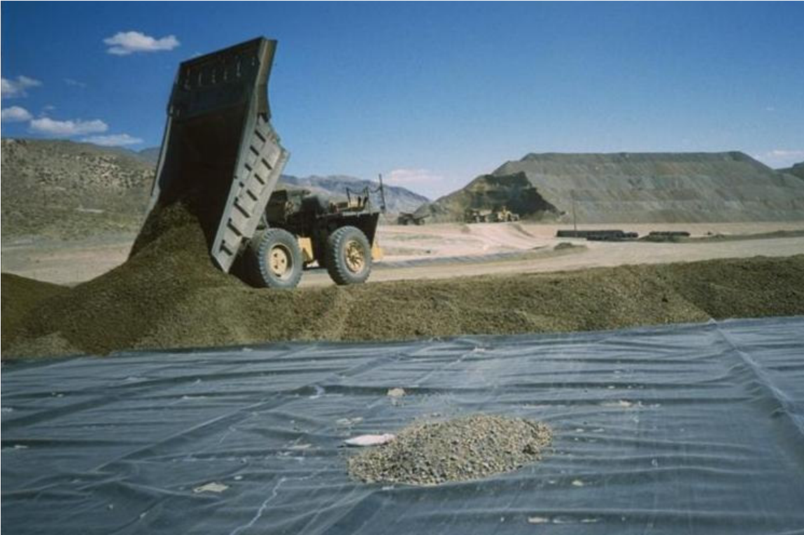
PHOTO 5 – DRAIN COVER FILL PLACEMENT ON THE PAD LINER SURFACE
