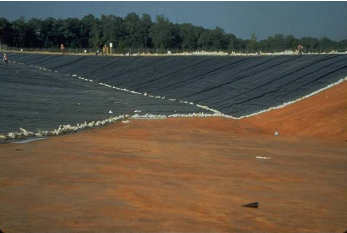
PHOTO 4 – COMPOSITE CLAYEY SOIL AND GEOMEMBRANE LINER SYSTEM
